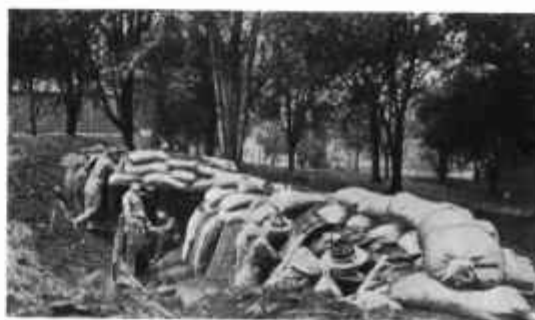
TRENCHES WITH WICKER WORK AND SAND BAGS
